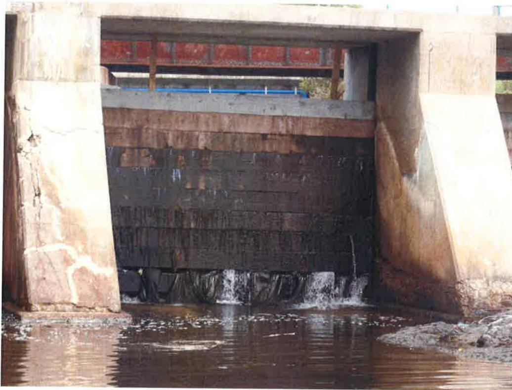
Blind River Dam September 2 – After leaks sealed gate 4
