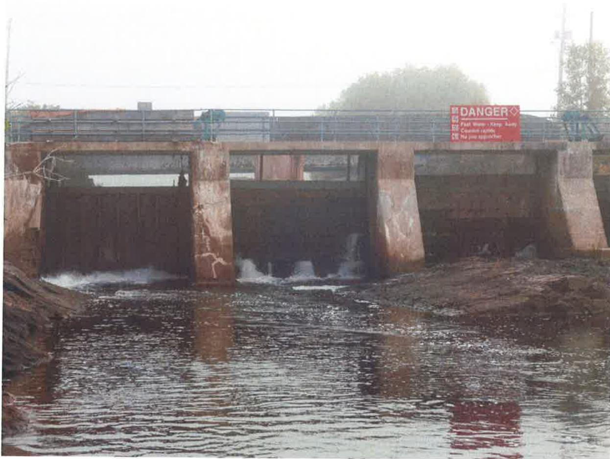
Blind River Dam August 2015 showing excessive leakage gates 4 and 5
