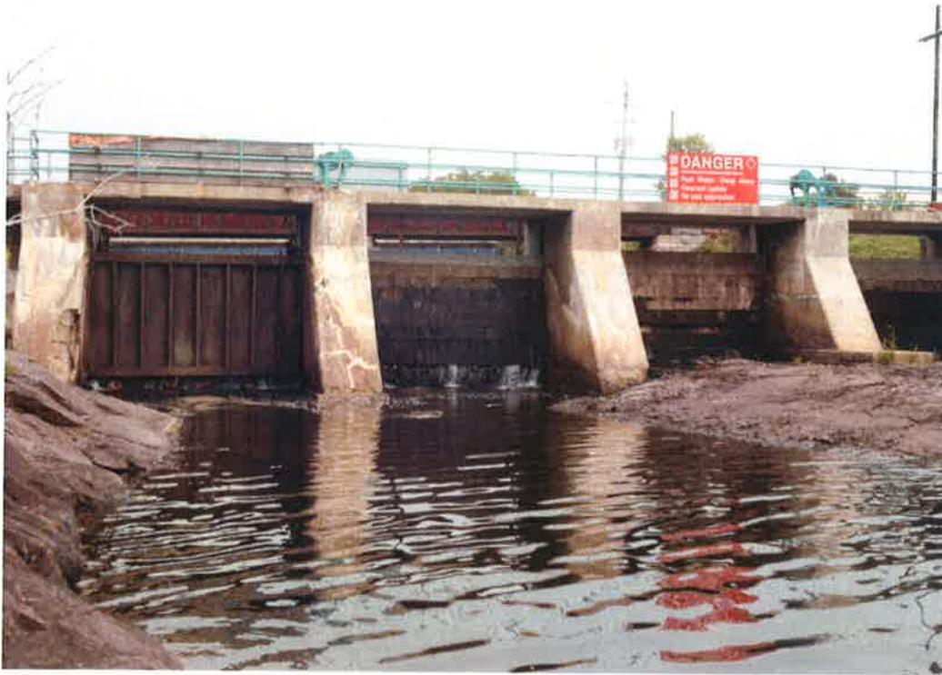
Blind River Dam September 2, 2015 after leaks sealed gate 3
