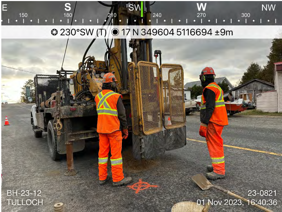
Photo 22: BH-23-12 during advancement. Photo taken facing southwest.
