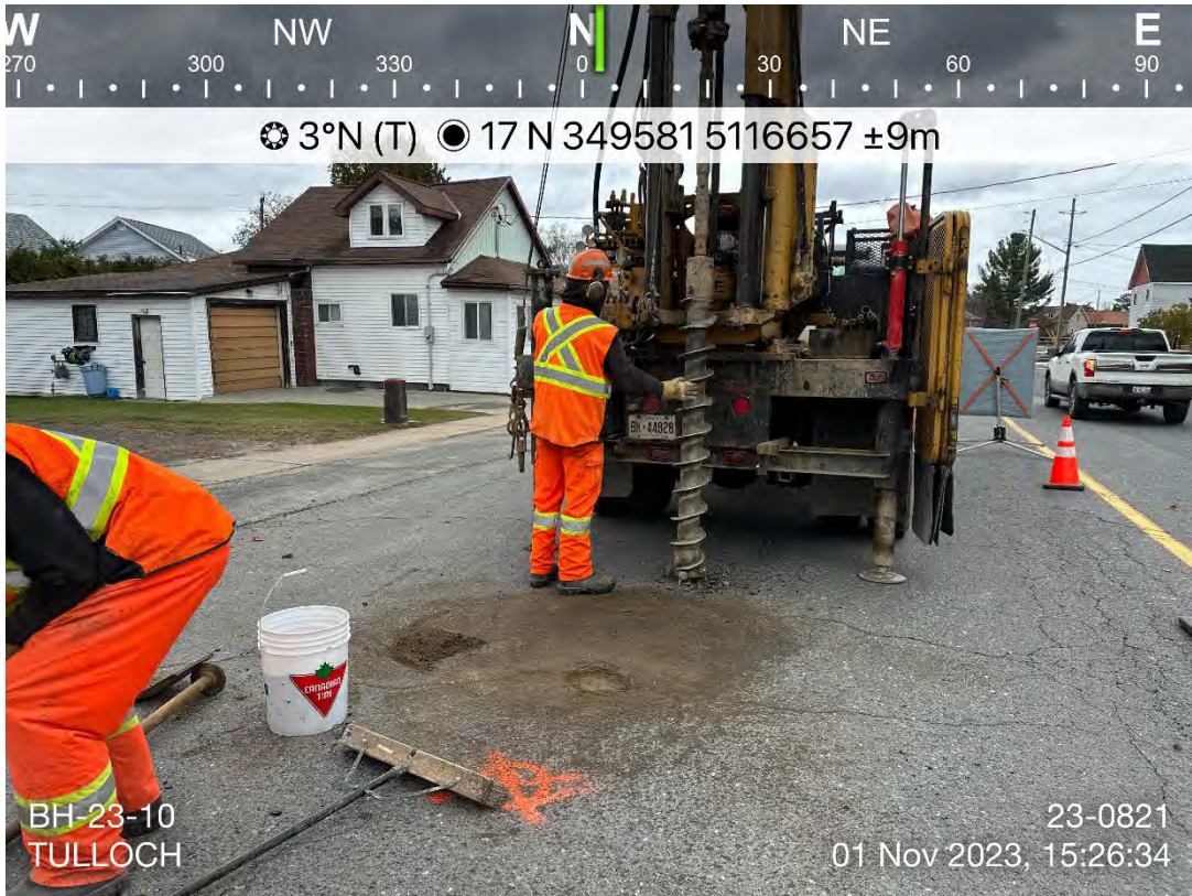
Photo 18: BH-23-10 during advancement. Photo taken facing north.
