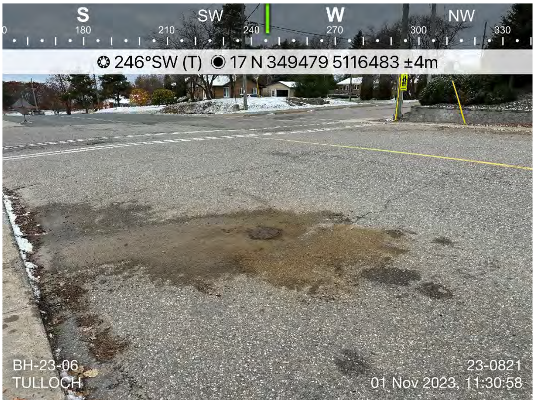
Photo 12: BH-23-06 following completion of backfill. Photo taken facing southwest.
