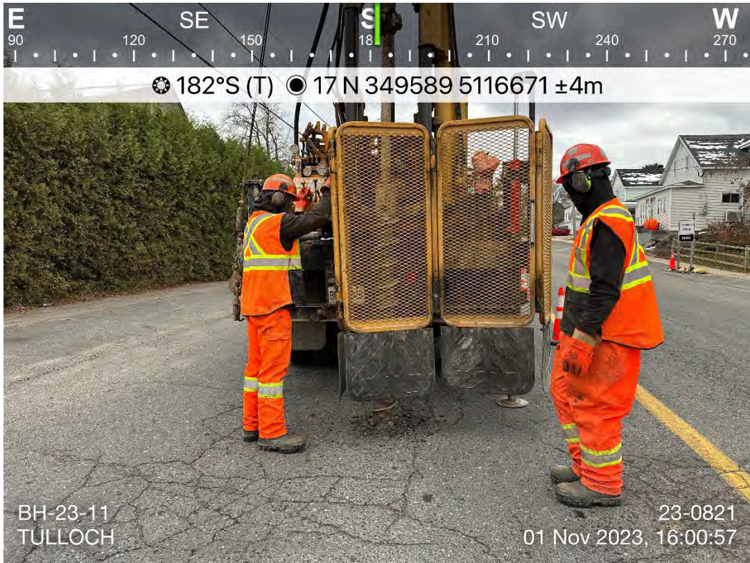
Photo 20: BH-23-11 during advancement. Photo taken facing south.
