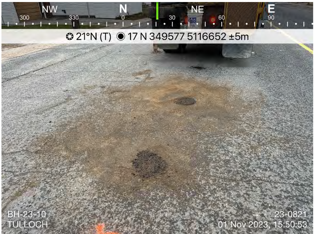
Photo 19: BH-23-10 following completion of backfill. Photo taken facing northeast.
