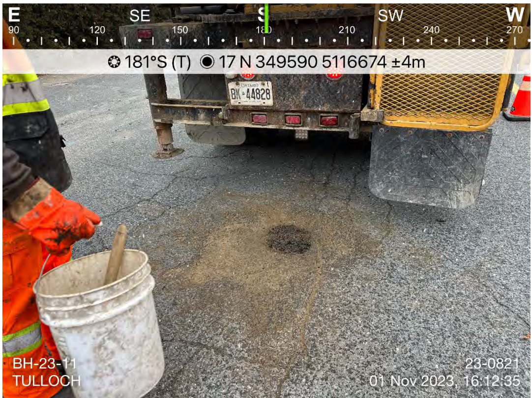
Photo 21: BH-23-11 following completion of backfill. Photo taken facing south.
