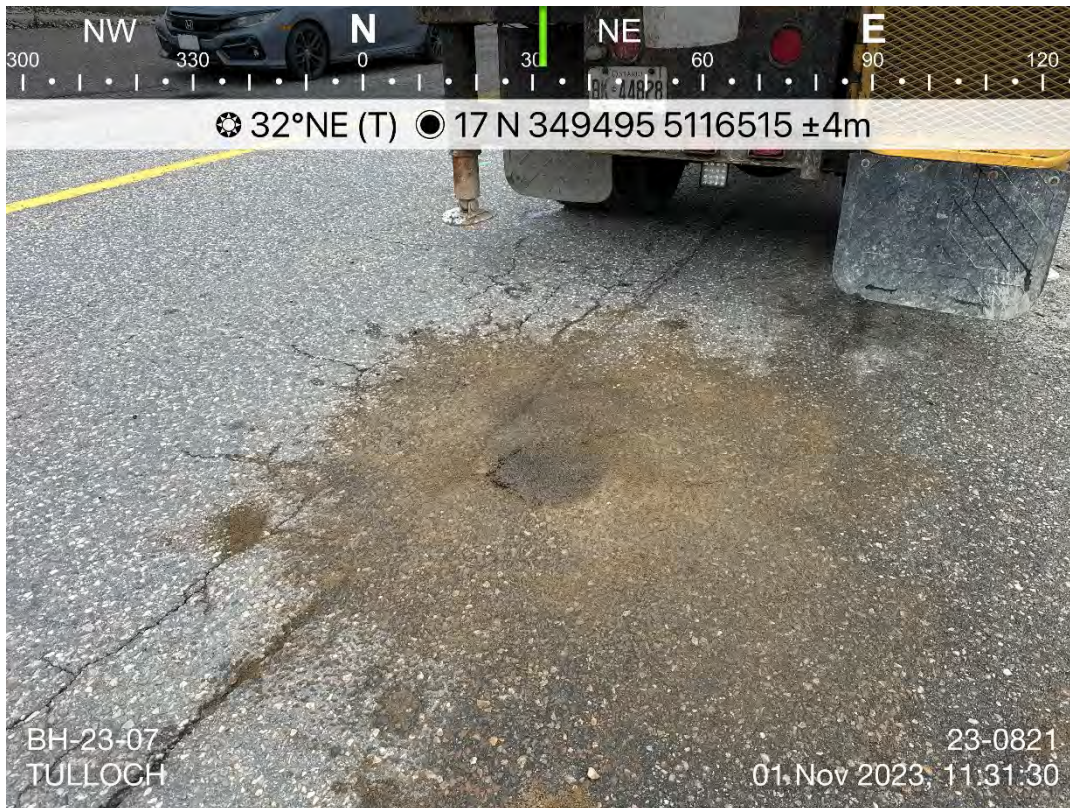
Photo 13: BH-23-07 following completion of backfill. Photo taken facing northeast.
