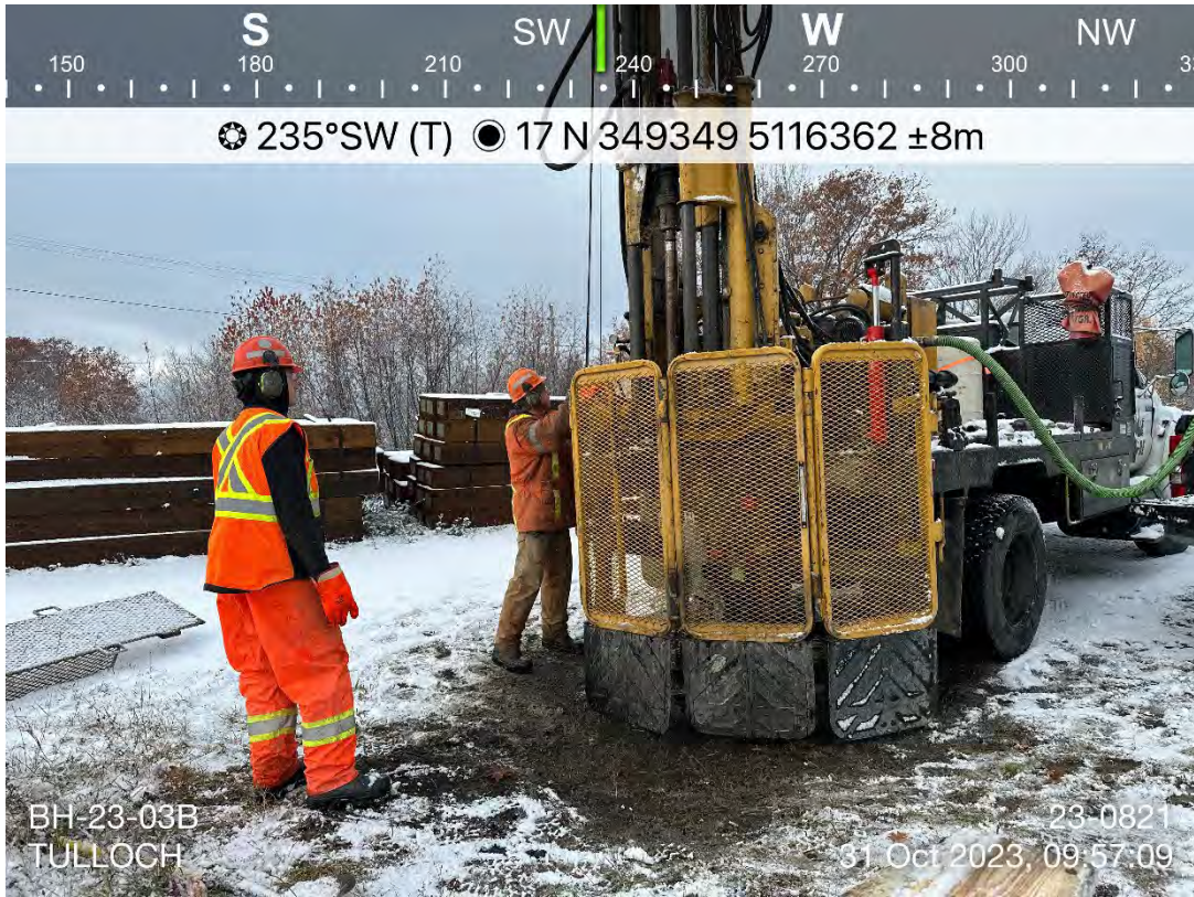
Photo 5: BH-23-03 during advancement. Photo taken facing southwest.
