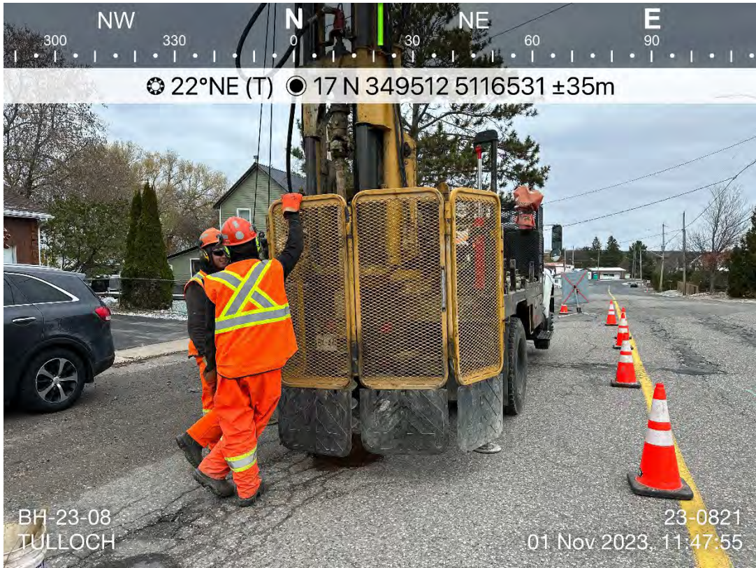
Photo 14: BH-23-08 during advancement. Photo taken facing northeast.
