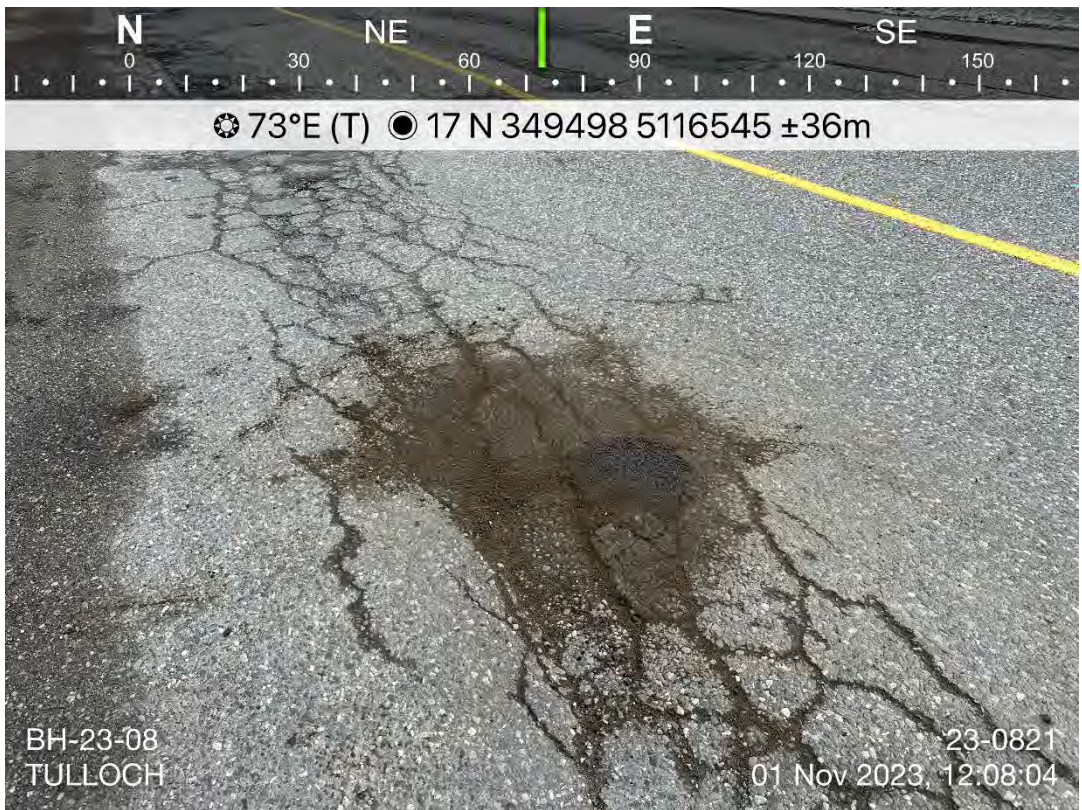
Photo 15: BH-23-08 following completion of backfill. Photo taken facing northeast.
