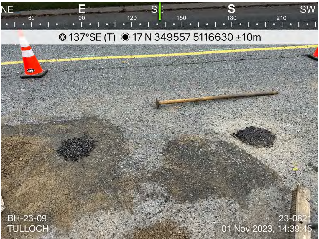
Photo 17: BH-23-09 following completion of backfill. Photo taken facing southeast.
