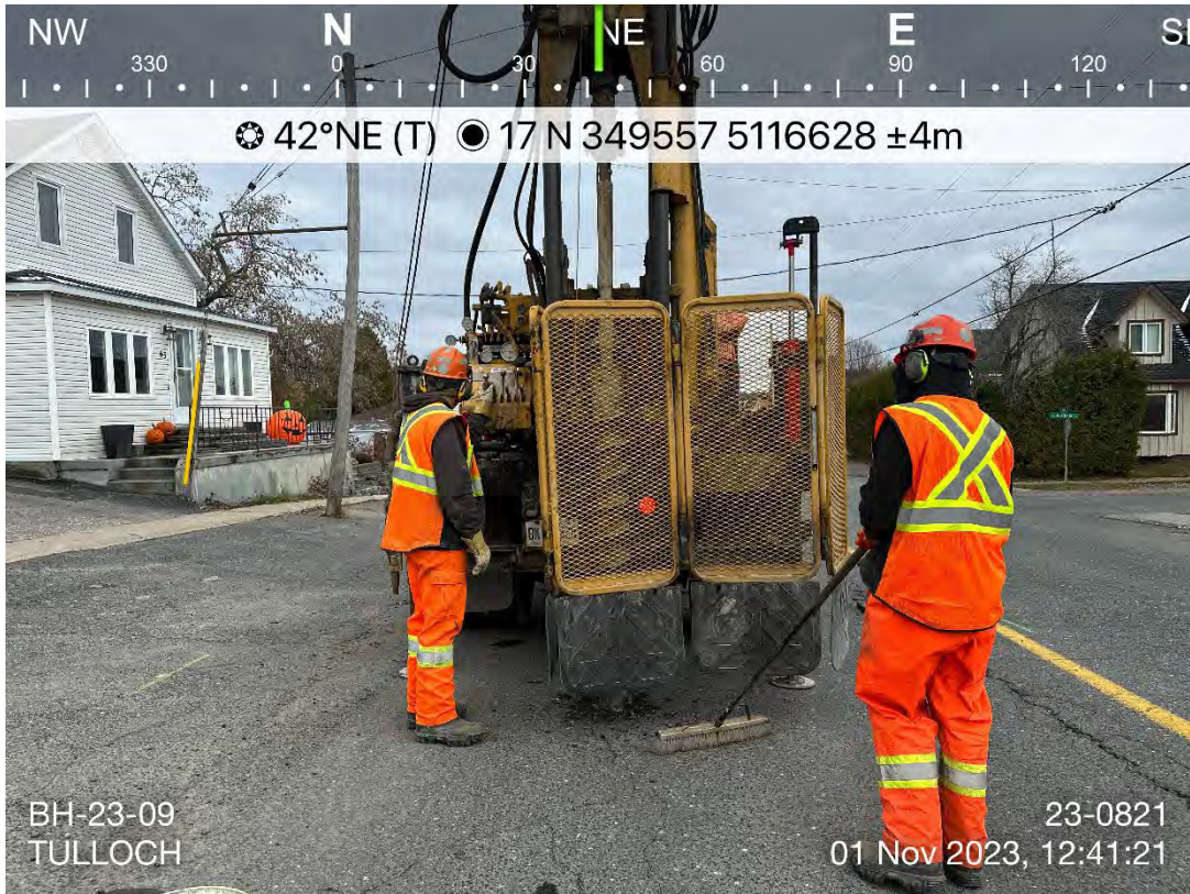
Photo 16: BH-23-09 during advancement. Photo taken facing northeast.
