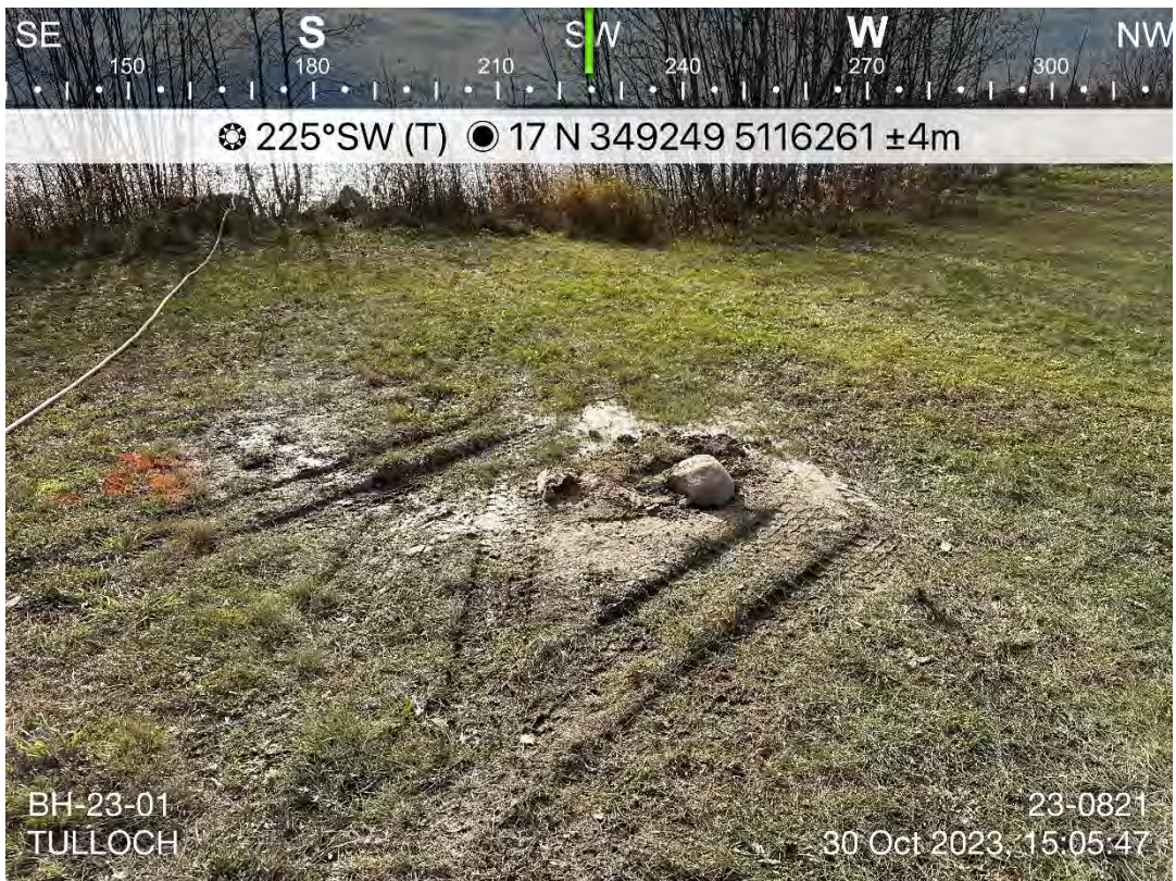
Photo 2: BH-23-01 following completion of backfill. Photo taken facing southwest.
