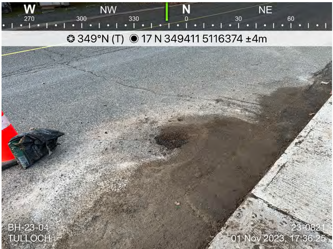
Photo 8: BH-23-04 following completion of backfill. Photo taken facing north.
