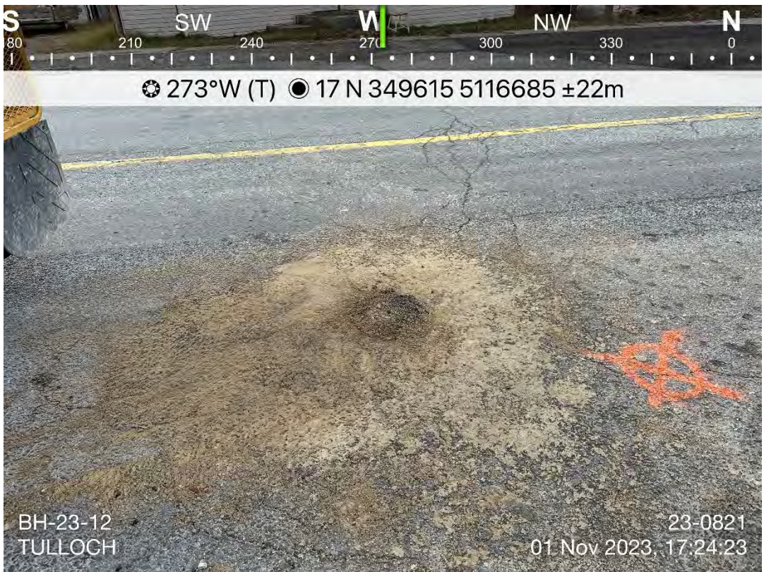
Photo 23: BH-23-12 following completion of backfill. Photo taken facing west.
