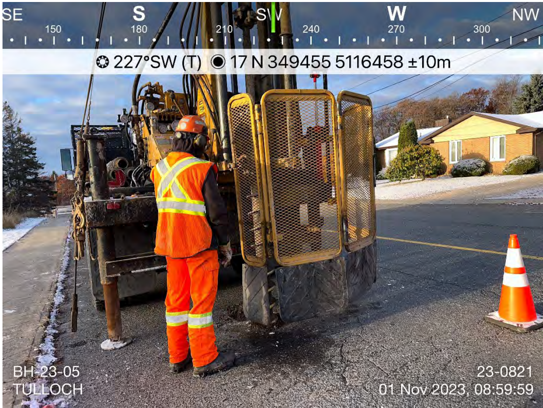
Photo 9: BH-23-05 during advancement. Photo taken facing south.
