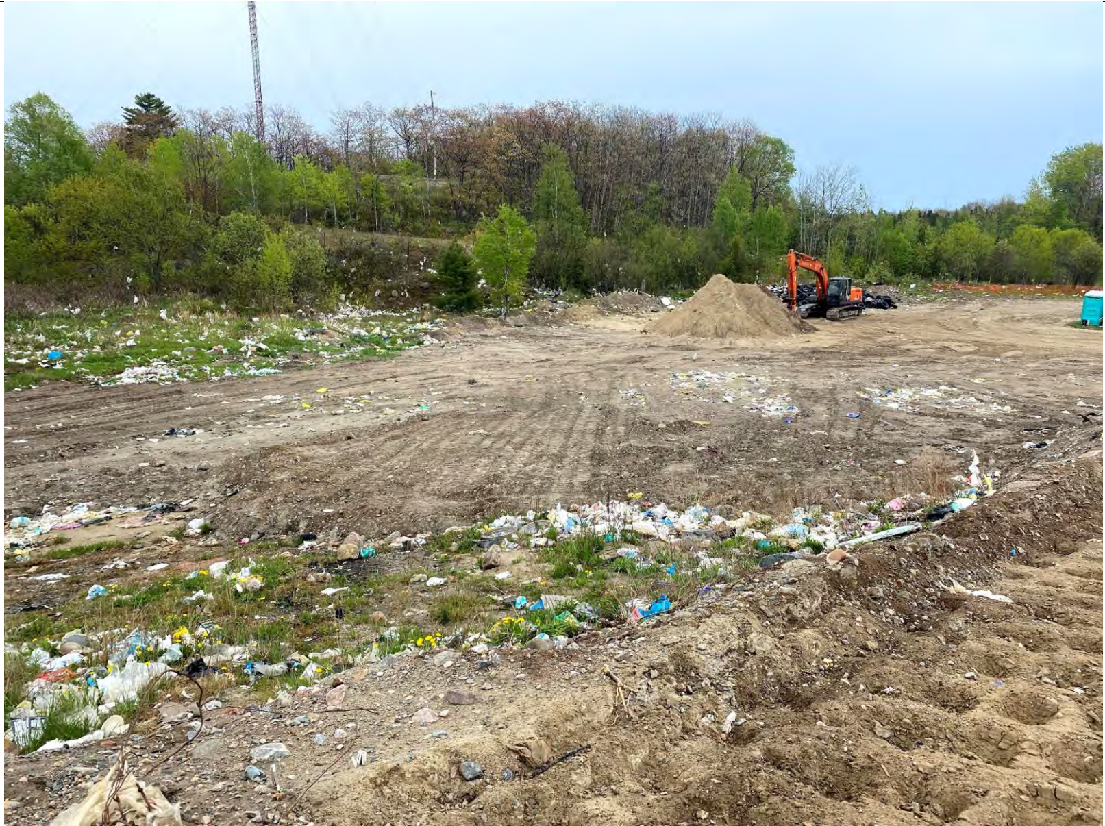
Photo 4 – Looking southeast from toe of landfill fill area
